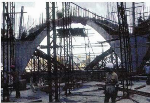
View showing newly concreted main arches
